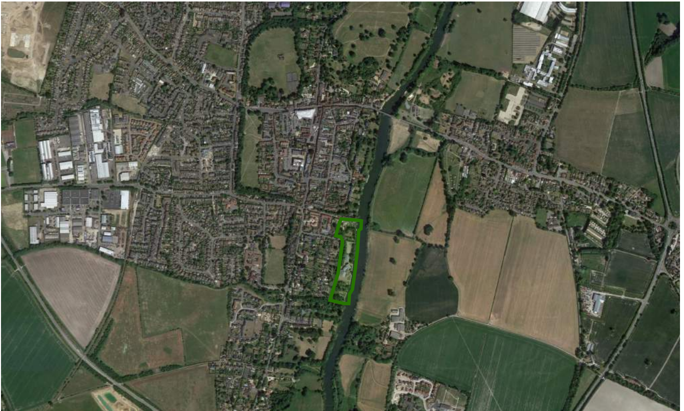
Figure 3: Approximate Location of Excluded Area (Site and Surrounding Land and Premises – Green Outline) Source: Google Maps with Williams Gallagher Mark Up
