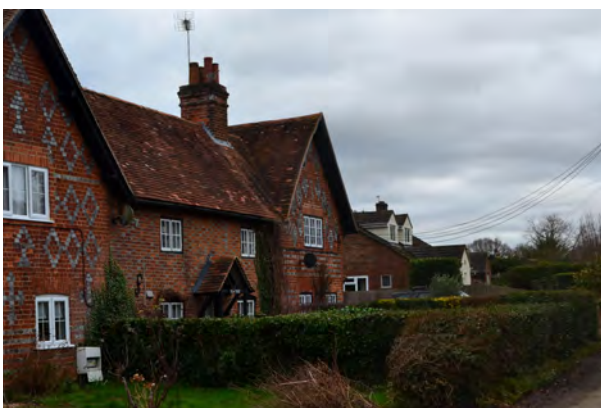
Photo 19: Cottages in view looking south-east on Gravel Road
