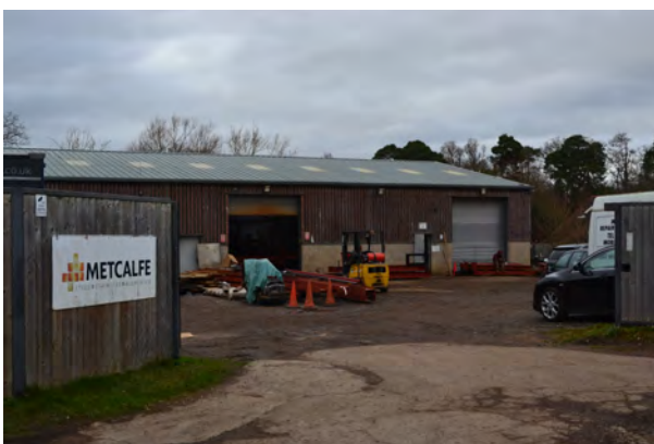
Photo 17: Industrial buildings, Dunsden Way
