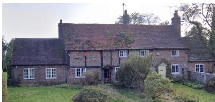
Figure 14: Jasmine and Timber Cottages are among the listed buildings in Crowsley
