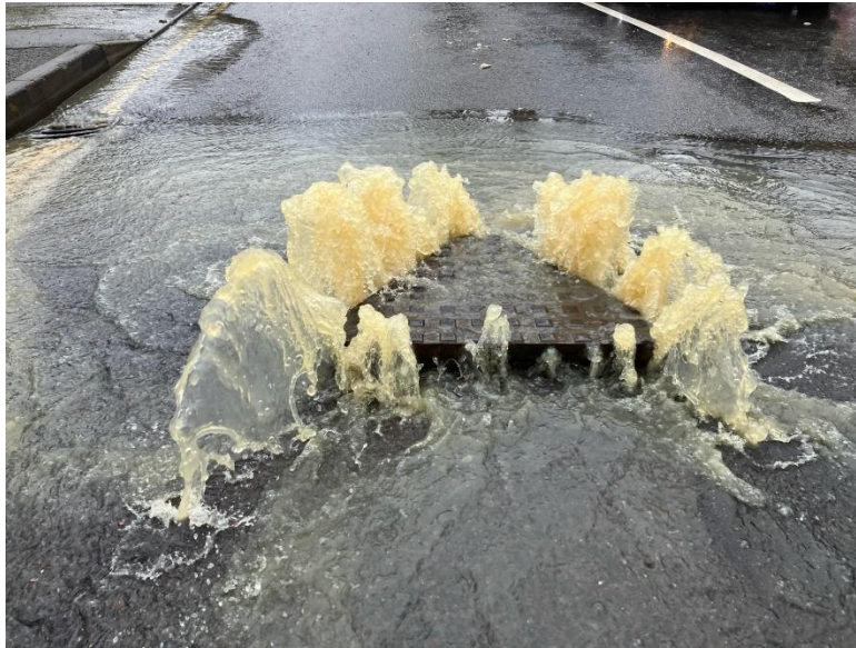
Flooding in the High Street caused by field run-off in nearby fields
