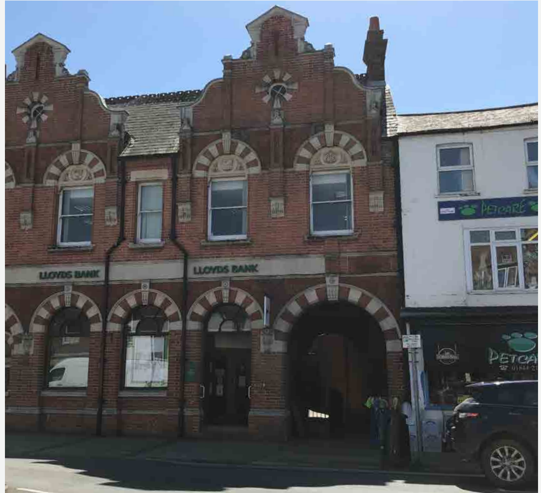
Figure 39: Grade II listed Lloyds bank building, built in 1890 in the Dutch style, Cornmarket
