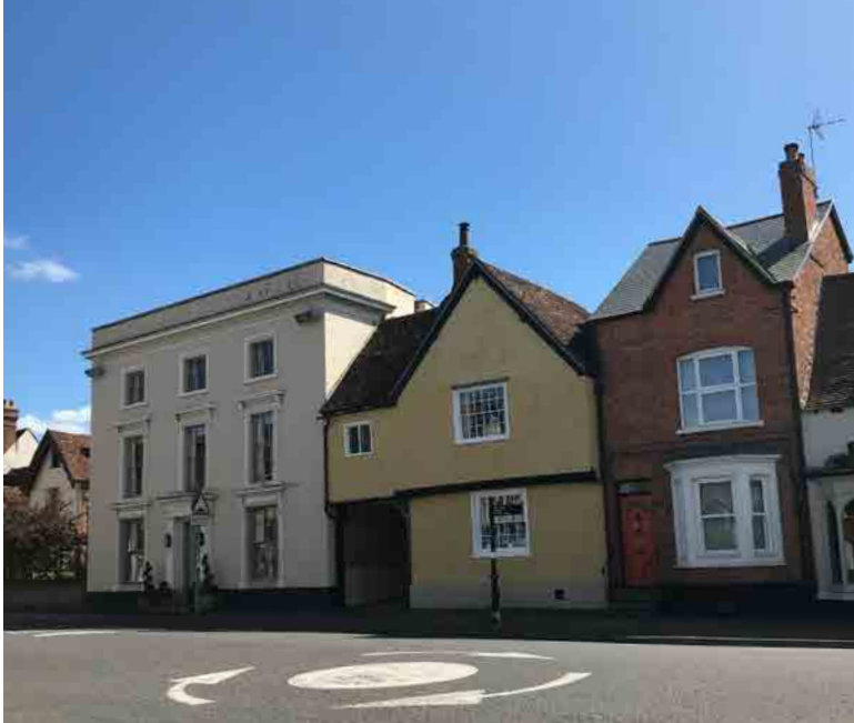
Figure 32: Northern end of High Street
