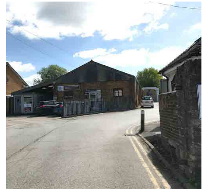
Figure 108: Site entrance, looking east
