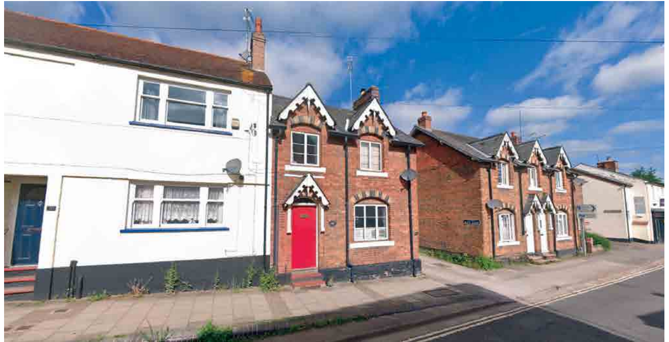
Figure 113: Victorian properties along North Street
