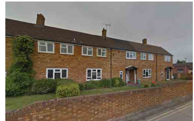
Figure 115: View east along Abingdon Close
