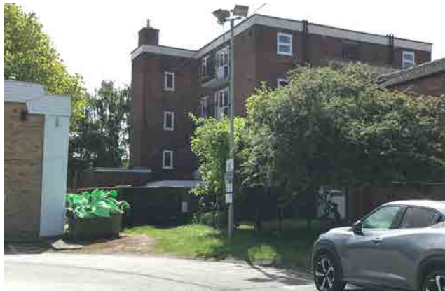
Figure 104: View east towards south eastern corner of the site
